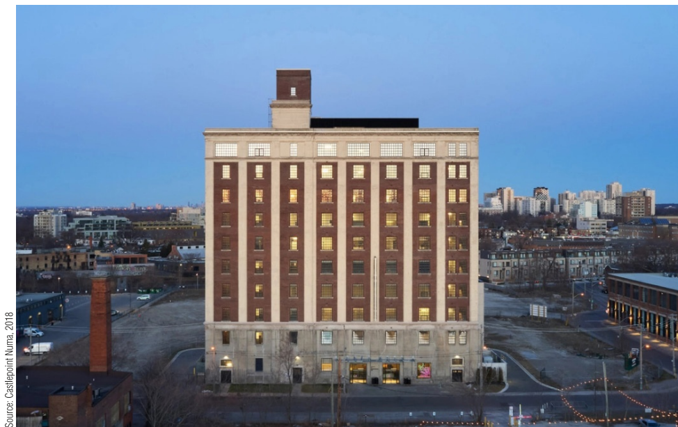
Figure 4: Tower Automotive Building and Surrounding site after completion of retrofit
