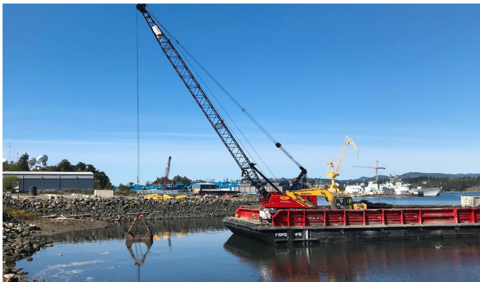
Figure 3: A dredging operation to remove contaminated sediment from the subtidal seabeds.
