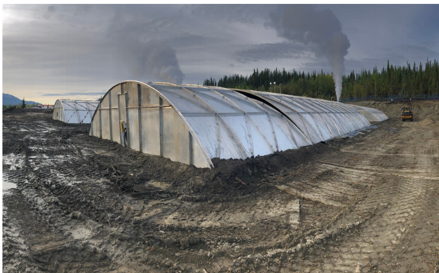
Figure 4. Image depicting the enhanced thermal conduction system used to treat contaminated soil at the Marwell Tar Pit.
