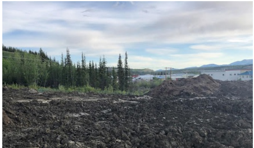
Figure 6. Image showing the site terrain at the beginning of remediation.
