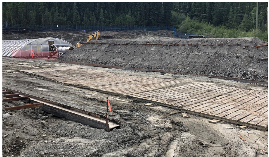
Figure 7. Image showing the storage and treatment of contaminated soil on-site.
