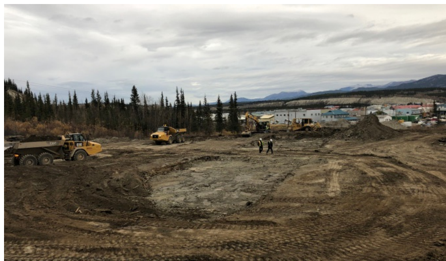
Figure 8. Image showing the site after excavation and prior to backfilling.
