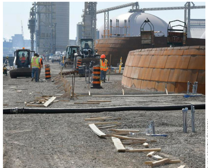
Figure 3: Construction Activities Occurring in the Summer of 2021.
