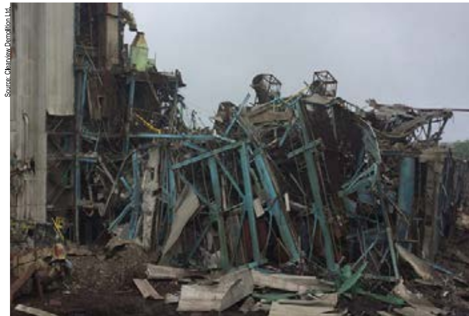
(fig.4) Demolition process leading to a 95% recycle rate.
